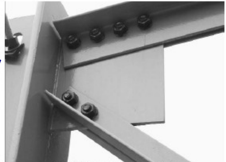
Figure 7-17. Misc. Connection: Truss Column C2 / Truss B7
