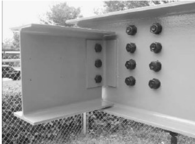
Figure 4-39. Shear Connection: Welded-bolted tee Girder B1 / Beam B1A
