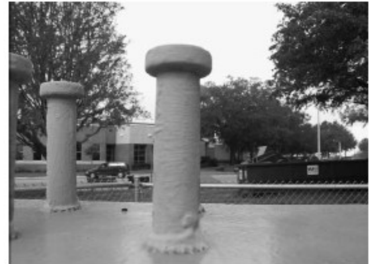
Figure 7-14. Misc Connections: Shear studs. Girder B1 / Shear Studs
