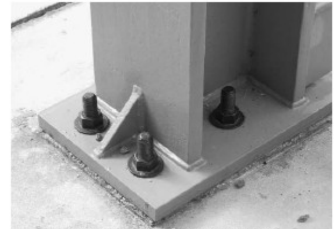
Figure 6-6. Column Connection: Base Plate Foundation / Column C1
