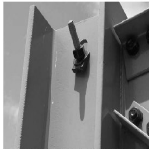
Figure 7-2. Misc. Connection: Clevis, plate & rod. Column C2 / Girder B6.
