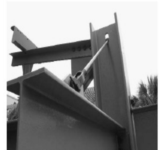
Figure 7-4. Misc. Connection: Clevis, plate & rod. Column C2 / Girder B6.
