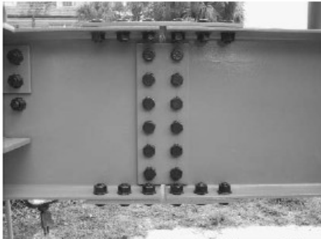
Figure 5-12. Moment Connection: All-bolted moment splice. Girder B3 / Girder B3
