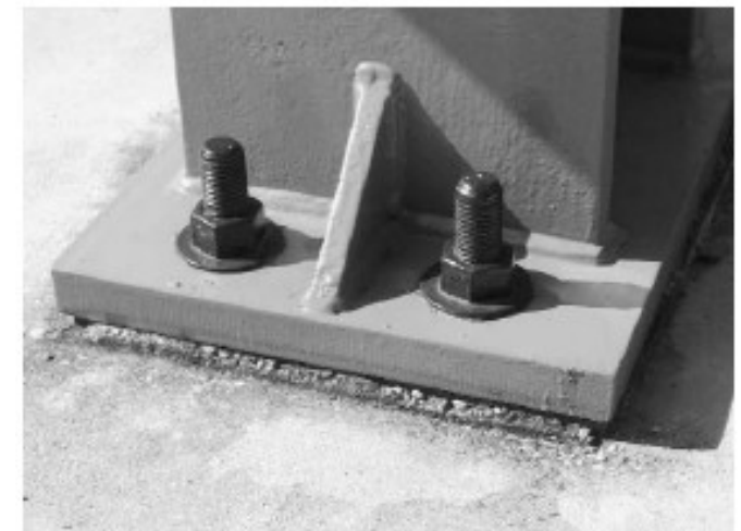
Figure 6-7. Column Connection: Base plate Foundation / Column C1
