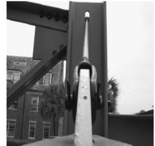
Figure 7-3. Misc. Connection: Clevis, plate & rod. Column C2 / Girder B6
