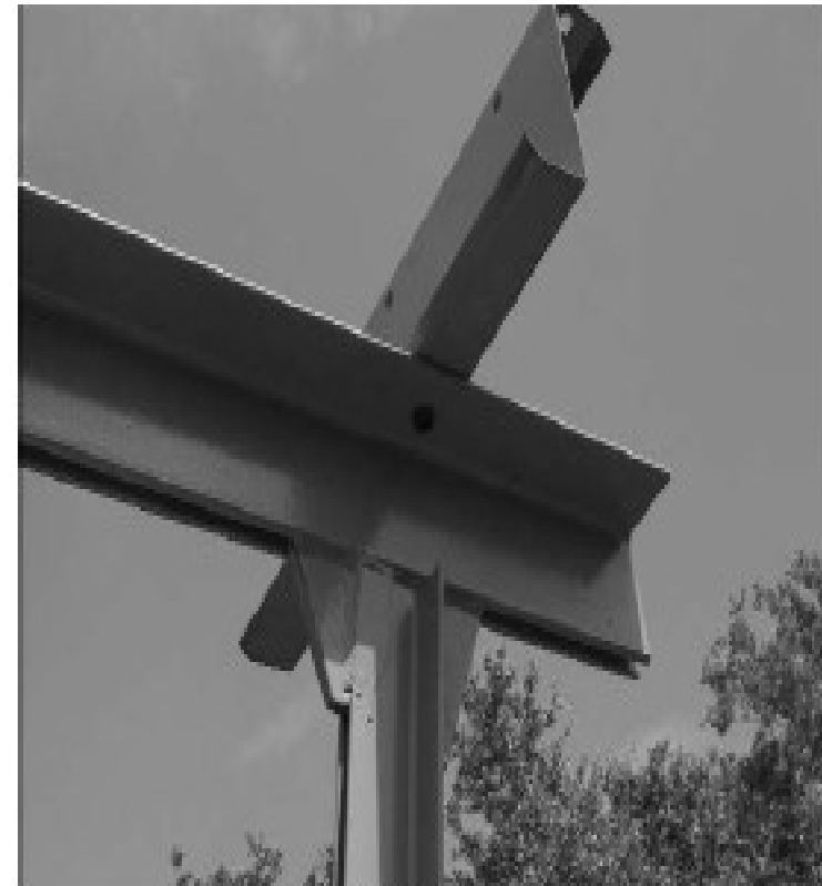
Figure 7-12. Misc. Connection: Z Purlin. Truss B7 / Purlin B9.
