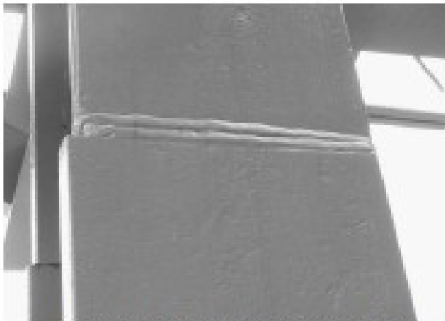
Figure 6-2. Column Connection: Column splice Column C1 / Column C2
