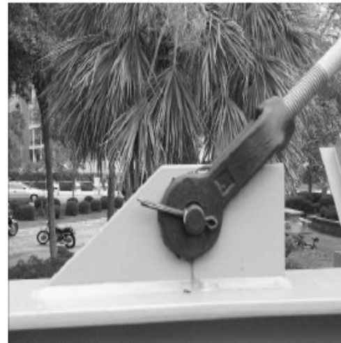
Figure 7-1. Misc. Connection: Clevis, plate & rod Column C2 / Girder B6
