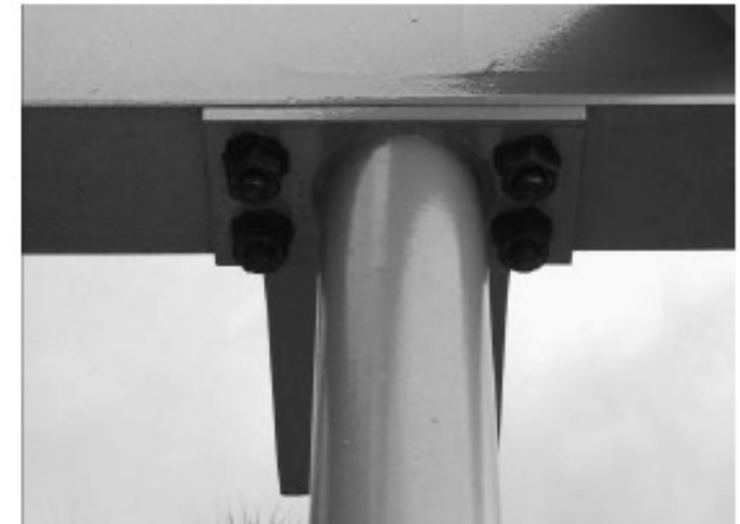
Figure 6-8. Column Connection: Base plate (bracing column) Girder B4 / Column C3 / Girder B8
