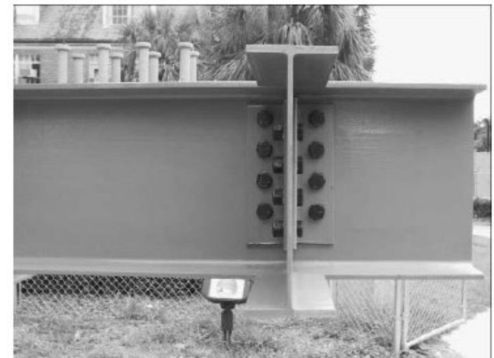
Figure 4-3. Shear Connection: All-bolted double angle Girder B1 / Beam B1B
