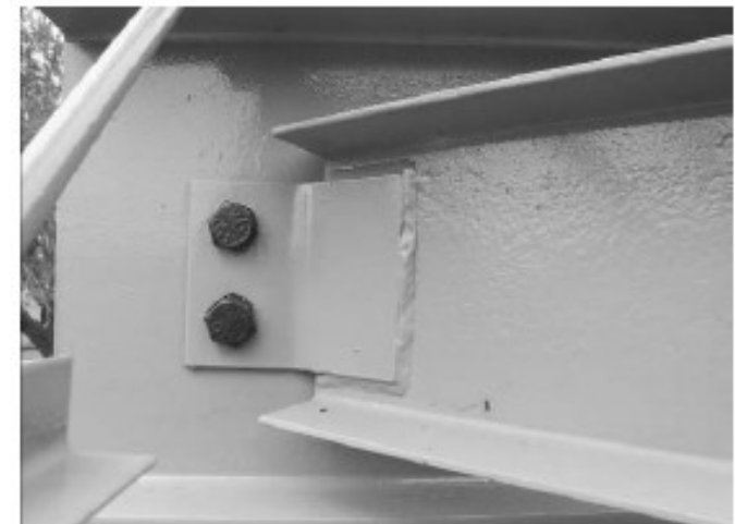
Figure 7-7. Misc. Connection: Bolted-welded bent-plate. Girder B5 / Beam B5A
