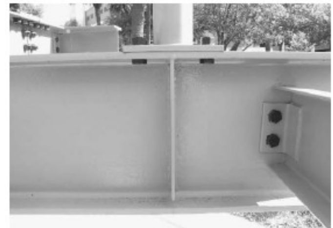
Figure 6-9. Column Connection: Base Plate (bracing column) Girder B4 / Column C3 / Girder B8
