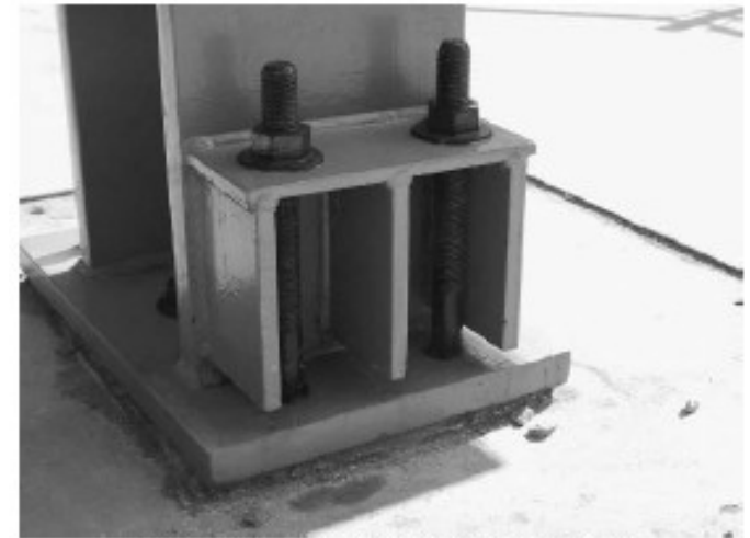
Figure 6-4. Column Connection: Base plate Foundation / Column C1
